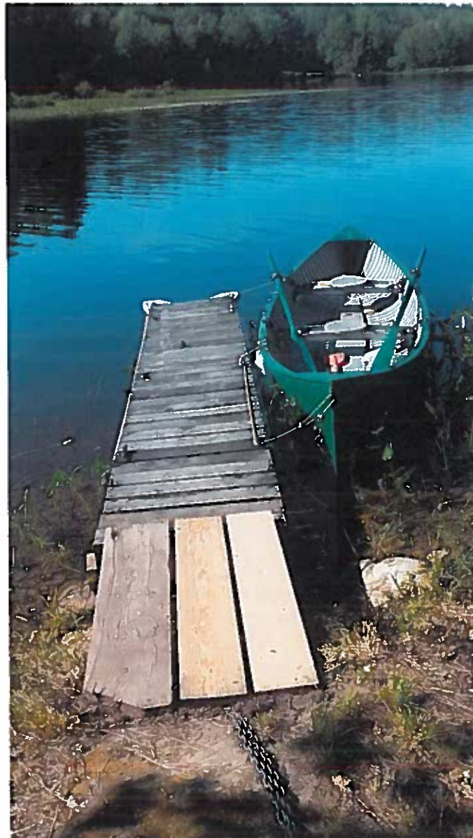
Stump Pond private dock installation
