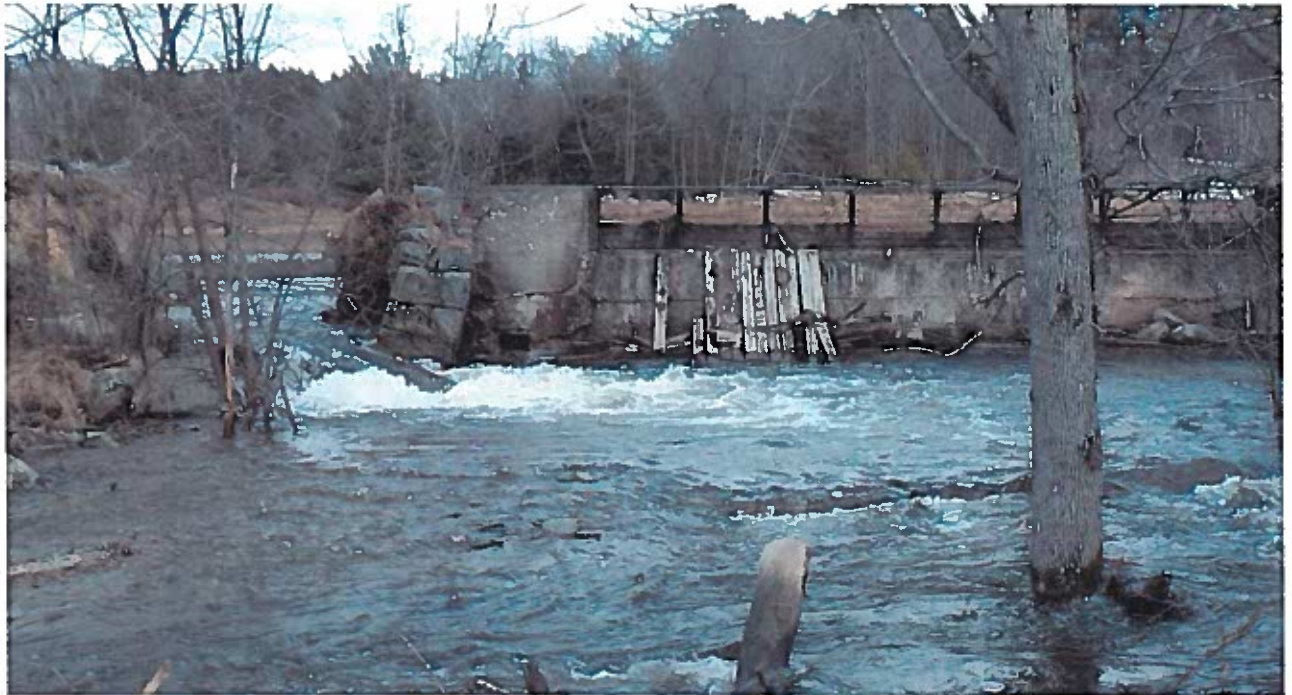
Haskell Dam Failure in 2020 due to Flood Flows
