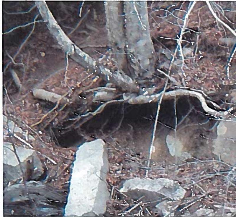
Typical shoreline or embankment erosion
