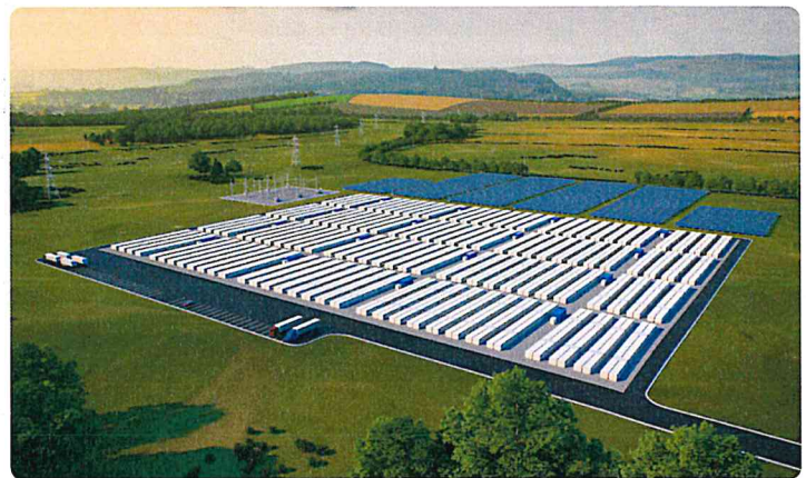
Rendering of a 56 MW Form Energy battery system
